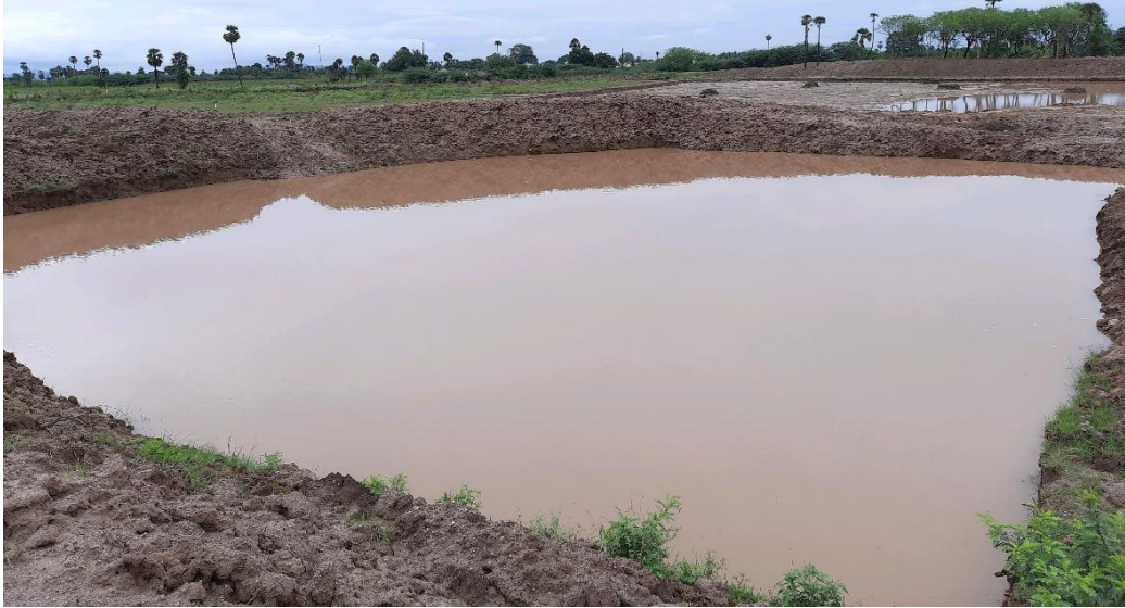
After uprooting of julifera and desilting of lake – rain water stored in the lake
