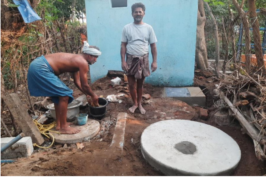
Converting single pit toilet into double pit.Total-24, Completed 12
