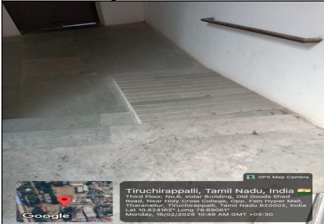
Ramp in Rehab Block
