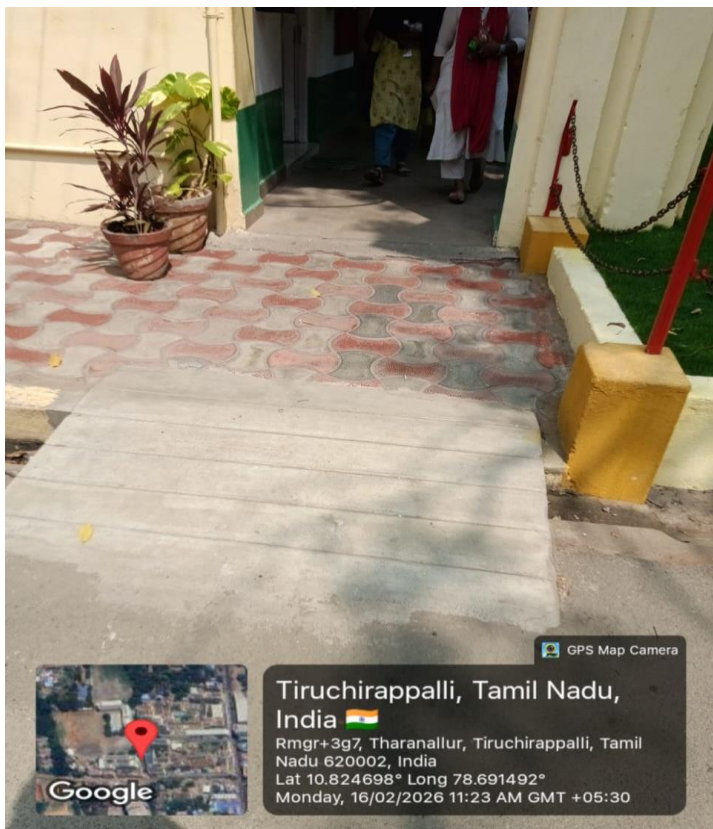
Ramp in Vice Principal Office
