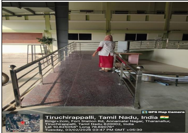
Ramp - Atrium Stage
