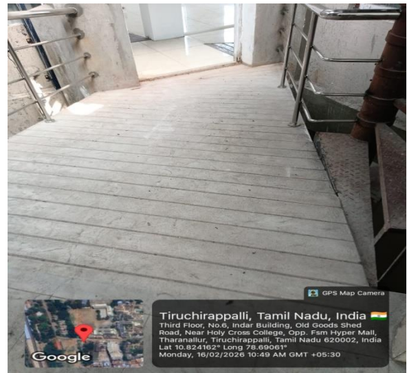
Ramp in Rehab Block
