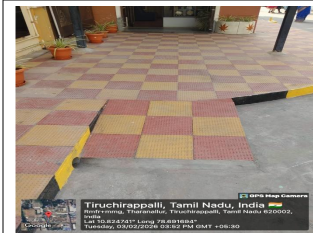
Ramp – Office Entrance
